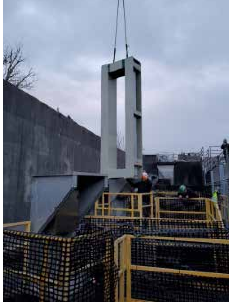
Figure 2. Installation of a slot antenna in Bonneville Dam Washington Shore serpentine weir (BO4). Image courtesy of Scott Livingston, PSMFC
