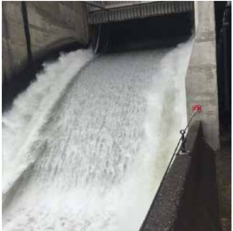
Figure 1. Lower Granite Spill Bay #1 with PIT tag detectors in operation and detecting tags May 2020. Photo courtesy of PTAGIS Staff
