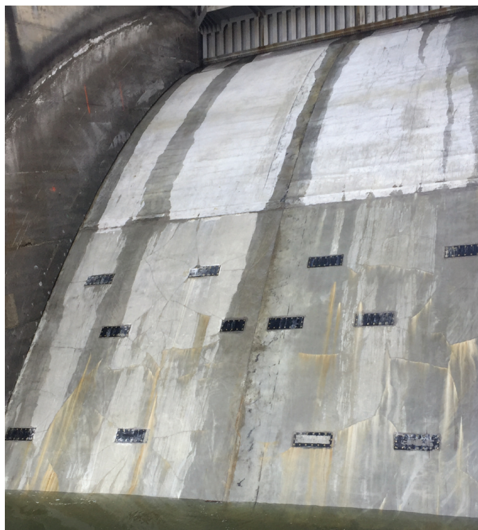
Image 2. Lower Granite Dam Spillway interrogation site displaying the black covers that allow access to antenna components for maintenance. Photo courtesy of PSMFC Staff
