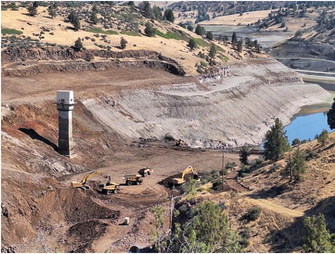
Klamath Dam Removals
