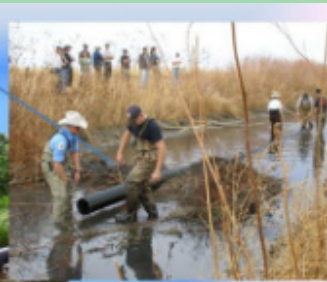
FLEXIBLE LEVELER: Single walled pipe & domed filter – Mike Callahan
