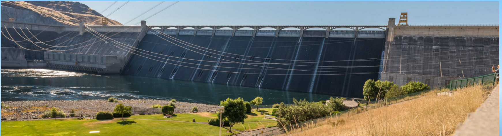
Grand Coulee Dam, Columbia River, Washington
