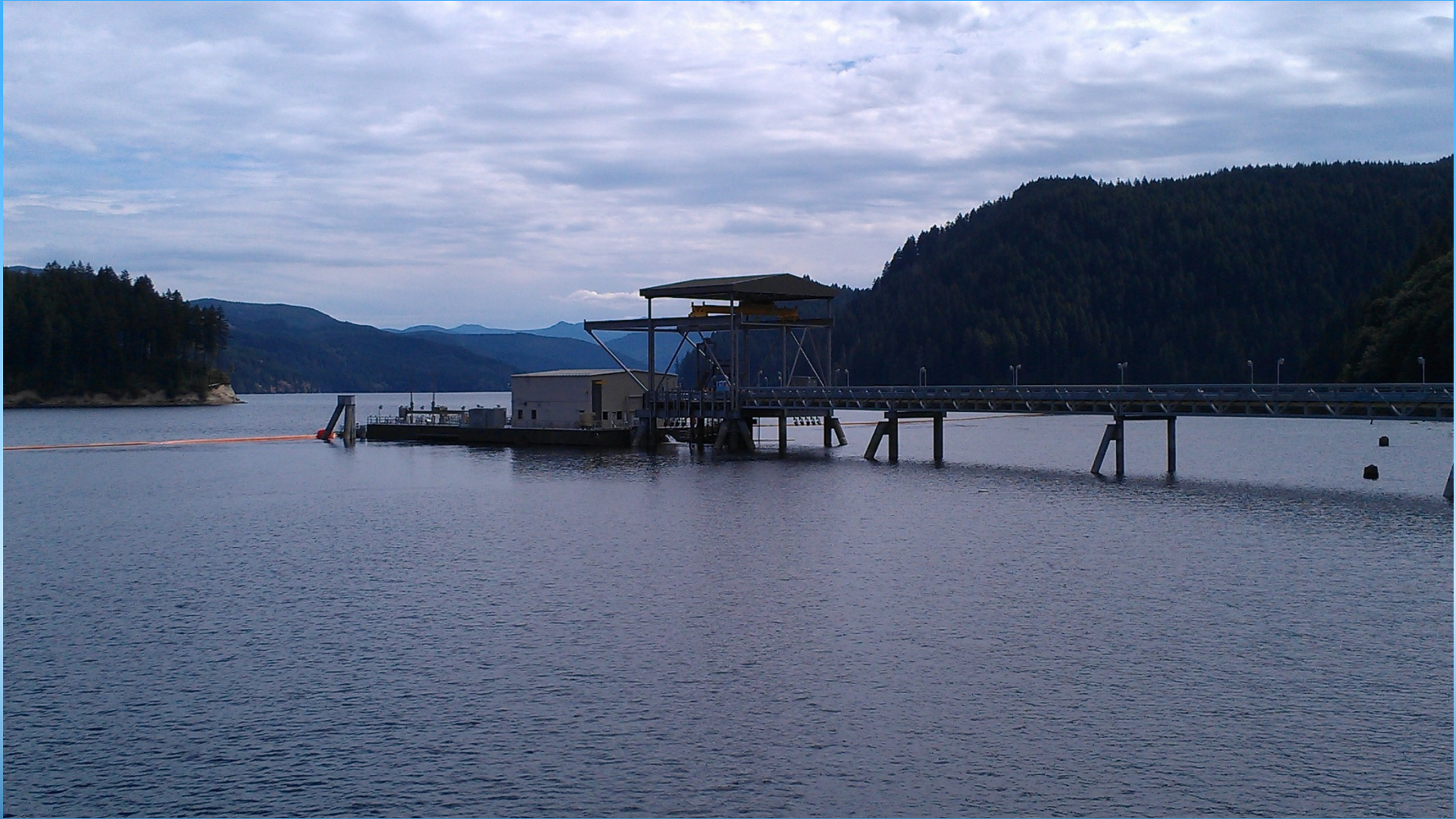
Swift Dam Fish Collector, Lewis River, Washington
