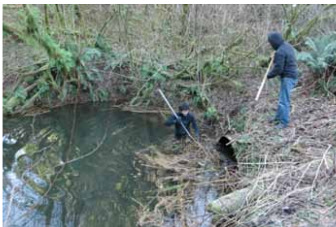
In preparation for installing a beaver deceiver (alternate dam site above the culvert), the existing plugged culvert is cleared.
