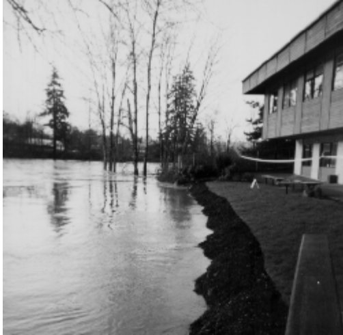
Figure 1. Floodwaters threatened PSMFC's Gladstone office during February 1996.
