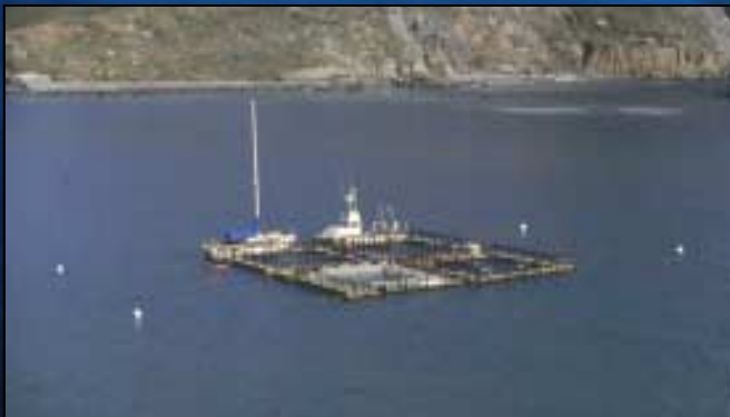
Catalina Island Cage Facility Catalina Island, CA System Capacity = 4 cages of 555 m 3 each
